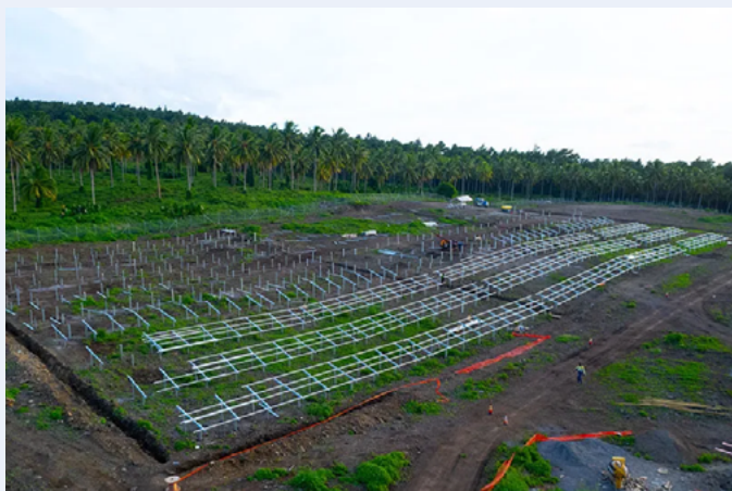
Construction of the 1MW grid-connected solar photovoltaic farm coupled with a battery energy storage system (BESS) on Taveuni
